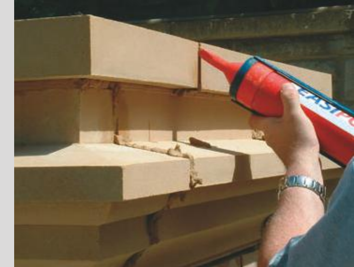
Easipoint mortar during installation.
